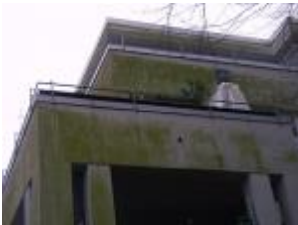
Image-No. 15 Explanatory facade that is infested with algae as presented in the ARD TV report Plusminus on 23.11.11)
